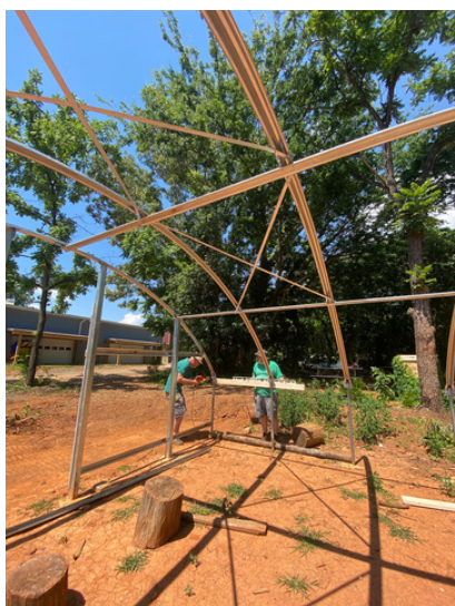
Mr. Chris and Mr. John attaching cross-braces to the greenhouse
